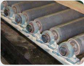
Overheating conveyor bearing
